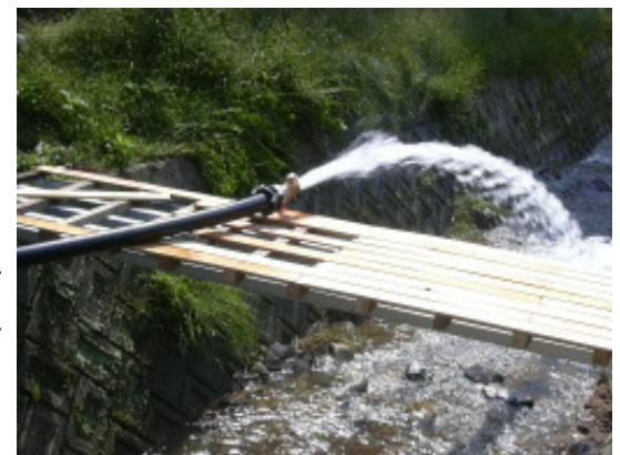
An air breather to eliminate air in the water. This can avoid hammering jet impact to the turbine.
