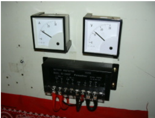
An ammeter (LHS), voltmeter (RHS) and a battery protector (below them). Our nominal output is about 120watts.
