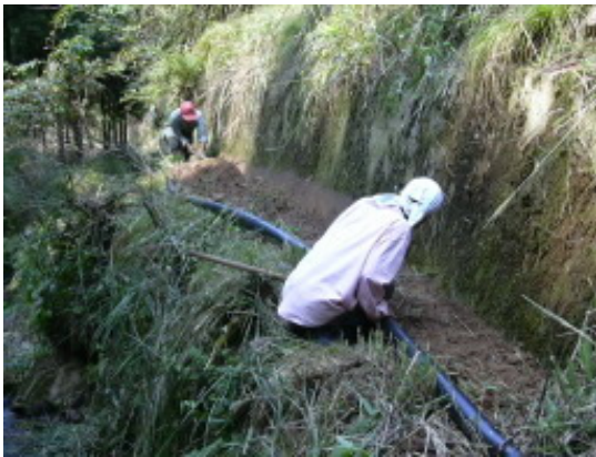
Penstock construction with owner's family.
