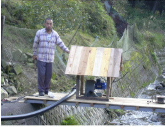
A power house (turbine & generator). The owner's son is a good carpenter.
