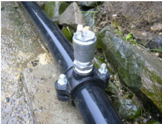
An air breather to eliminate air in the water. This can avoid hammering jet impact to the turbine.
