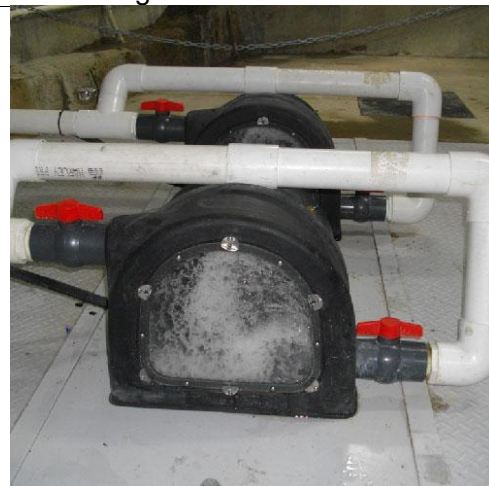
Manifold assembled on turbine
