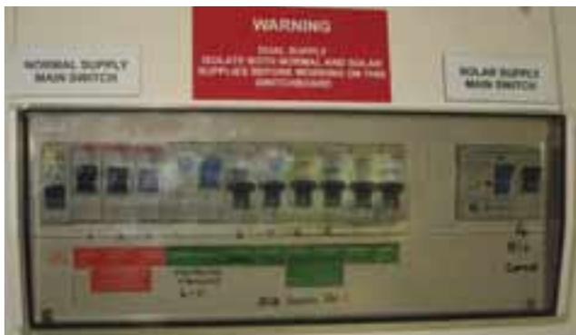
not operate tag' on the circuit breaker or physically isolate the battery bank by removing the battery cabling, first from the negative
