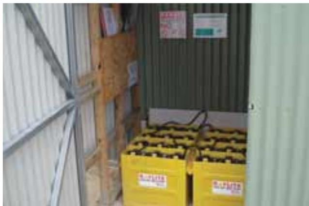
The batteries should be located in accordance with manufacturer's recommendations. The battery bank must be protected by a suitable enclosure which is only accessible by appropriately authorised people (eg. system owner, installer, service person). In large sheds the battery bank should still be housed in either a separate room or battery box to prevent unauthorised access and to separate spark sources
