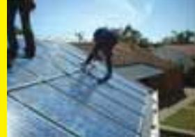
In most situations cleaning is only necessary during long dry periods when there is no rain to provide natural cleaning. To remove a layer of dust and dirt from the modules, simply wash the module with water. If the module has thick dirt or grime, which is harder to remove, wash with warm water and a sponge. Washing the modules is similar to washing glass windows but detergents should not be used. The modules should be cleaned when they are not excessively hot, typically early in the morning.
