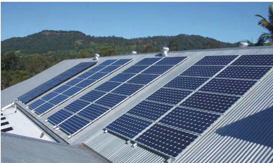
The most common maintenance task for solar modules is the cleaning of the glass area of the module to remove excessive dirt.
