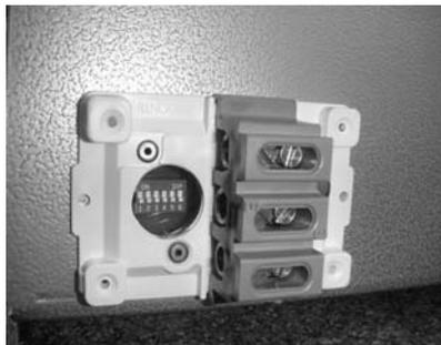
Settings are adjustable via DIP switches located inside the **Generator Input Junction Box**.
